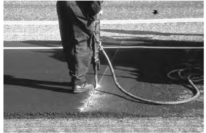
FIGURE 17-2 Removal of material at butt joint.
