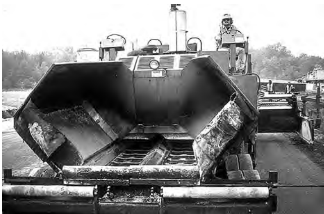
FIGURE 15-4 HMA paver with wings lifted.
