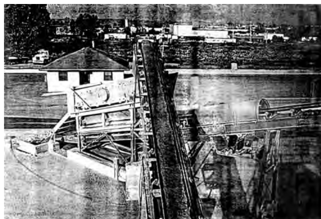
FIGURE 6-8 Double-deck scalping screen on drum mixer with air-operated deck selector.
