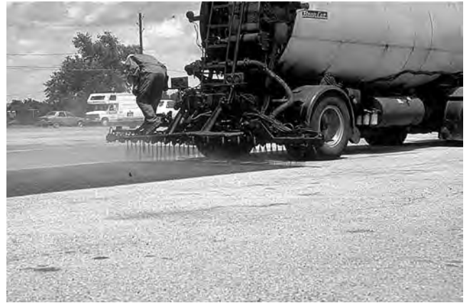
FIGURE 14-7 Distributor applying tack coat.
