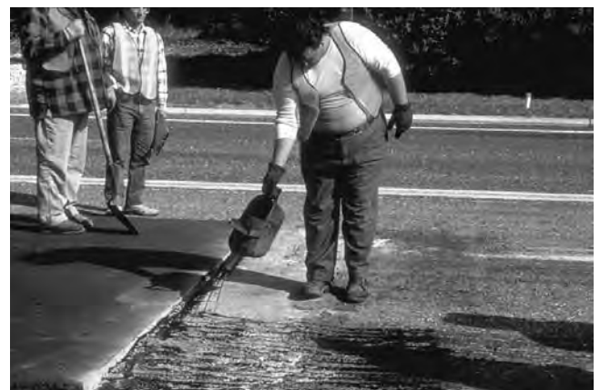
FIGURE 17-3 Application of tack at butt joint.
