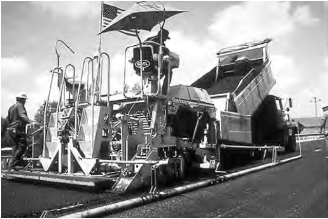
FIGURE 16-4 Paver with mobile reference employing rigid pipe.
