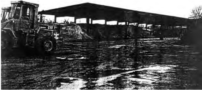
FIGURE 6-1 Covered aggregate stockpiles.
