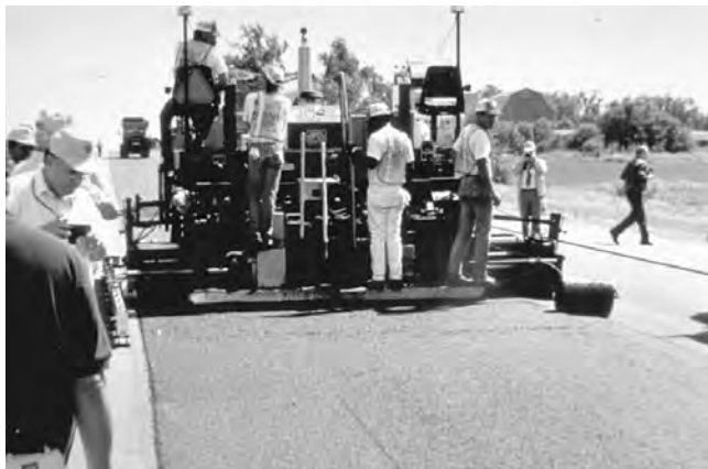
FIGURE 17-17 Compaction of mix in wedge joint.
