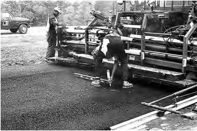
FIGURE 16-11 Checking slope of mat surface behind paver.
