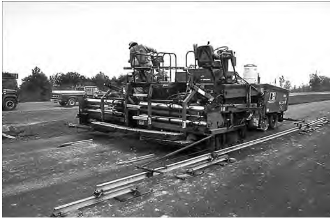
FIGURE 16-6 Floating-beam mobile reference with shoes at ends of beam.
