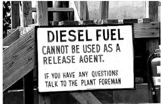
FIGURE 13-6 Diesel fuel is an unacceptable release agent.
