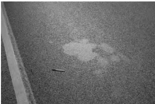
FIGURE 19-9 Fat spot caused by fuel oil spill prior to overlay construction.
