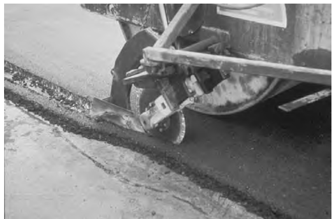
FIGURE 17-11 Cutting wheel used to construct longitudinal joint.
