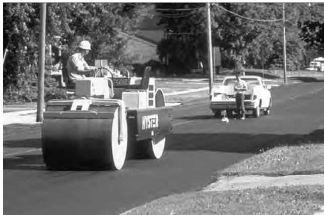
FIGURE 18-3 Static steel wheel roller.
