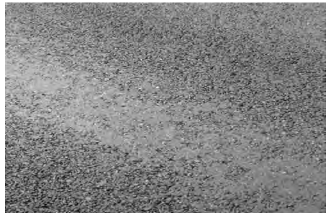
FIGURE 19-1 Nonuniform mat texture after compaction.
