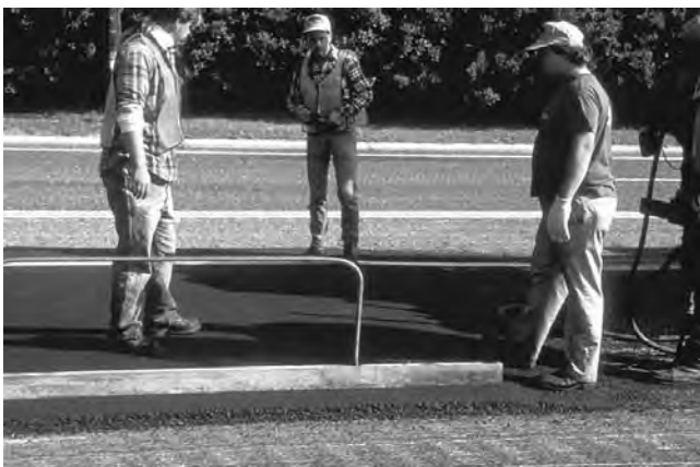
FIGURE 17-8 Checking smoothness at transverse joint.
