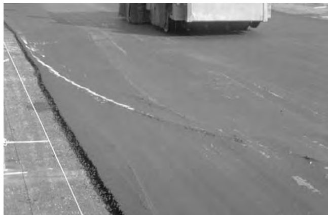
FIGURE 19-10 Roller marks in freshly laid asphalt pavement.
