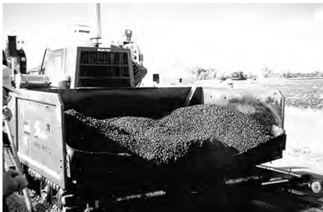
FIGURE 15-2 Loaded HMA paver hopper.
