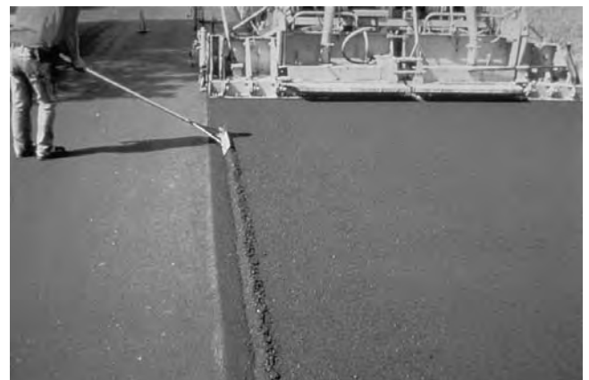
FIGURE 17-13 Raking of longitudinal joint.
