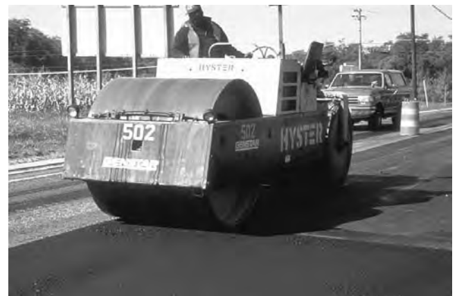
FIGURE 17-10 Longitudinal rolling of transverse joint.
