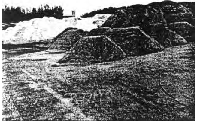
FIGURE 6-2 Horizontal stockpiles.
