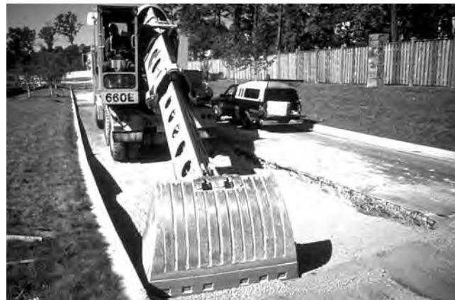
FIGURE 14-2 Removal of existing pavement prior to patching.
