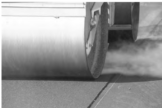
FIGURE 17-16 Compaction with edge of equipment inside longitudinal joint.
