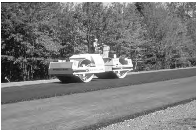
FIGURE 18-6 Vibratory steel wheel roller.
