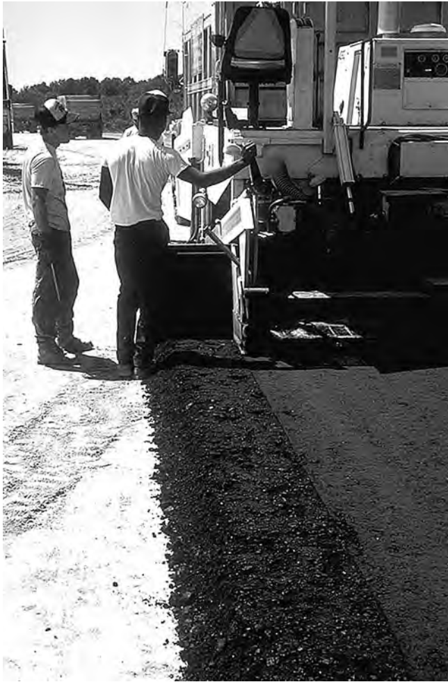
FIGURE 15-19 Difference in texture under strike-off extension.
