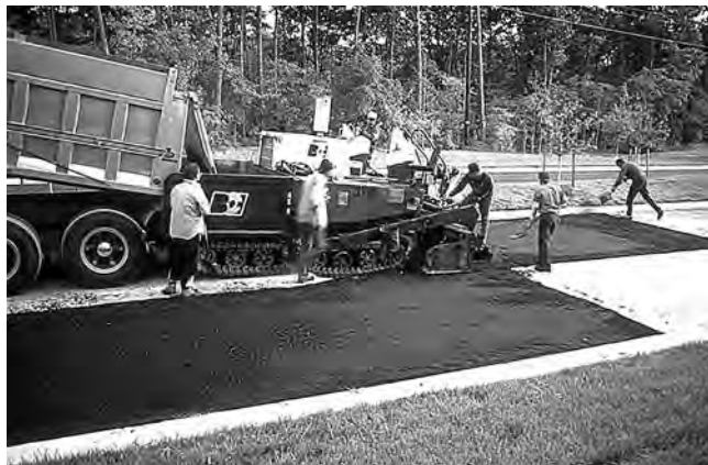
FIGURE 14-1 Patches placed with paving machine.
