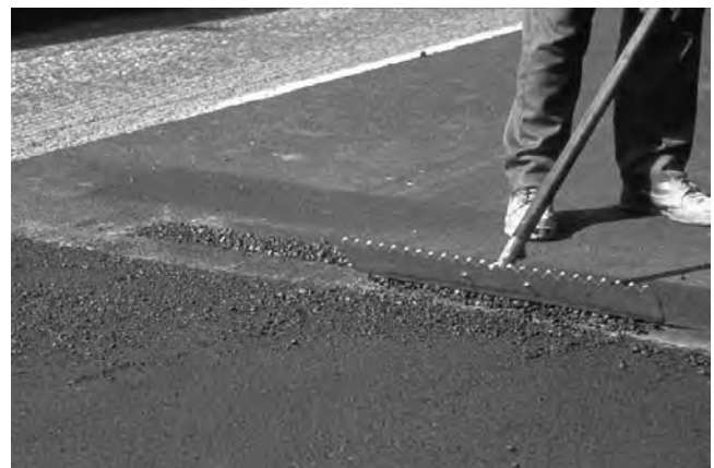
FIGURE 17-6 Raking of transverse joint.
