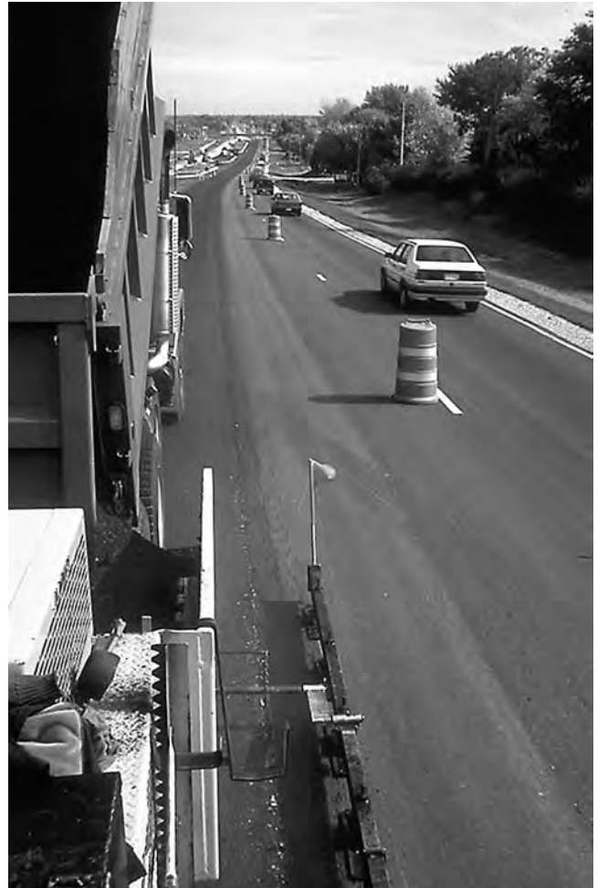
FIGURE 16-5 Floating-beam mobile reference.
