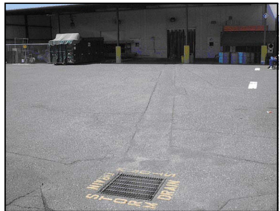
Figure 12. In addition to employee training, labeling storm drains is a good measure to educate employees.
